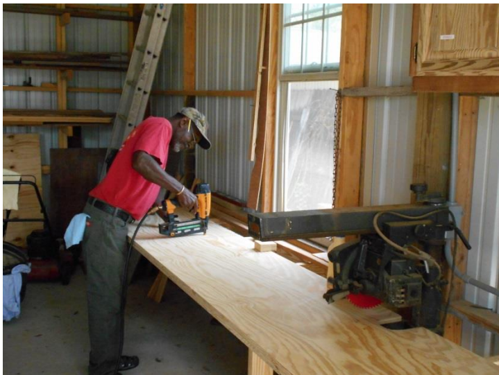
With the support frame in place, the saw is now put into position and two layers of \frac{3}{4} " plywood are attached using glue and nails.
