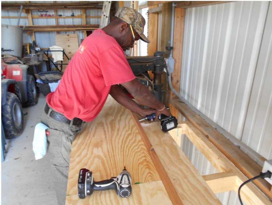
Next Alvin attaches the fence to the back edge of the top layer of plywood. No glue here, just screws, in case it ever has to be replaced.
