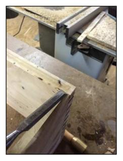
Using a sharp chisel I squared up the rounded ends left by the router in the stop rabbets. Notice the protrusion of the dovetail joints. I will clean those up once I am sure of everything being square and tight.
