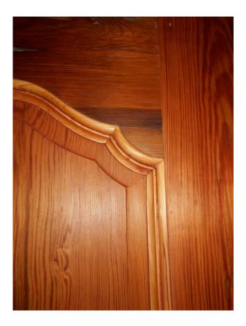
With the molding in place on one side, the panel is then put in place and the molding is fitted to the opposite side. The photo at right shows the completed upper right corner with the finish applied. The intent with the finish is to make the door look as though it's been around for awhile.
