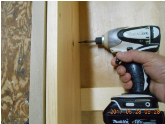
Attaching with screws from inside the drawer and the bottom two fronts attached. This set of cabinets will be painted white and installed in a large closet. They are constructed of birch plywood, poplar and white pine for the drawer boxes. I hope that in reading this you have found it to be of helpful.
