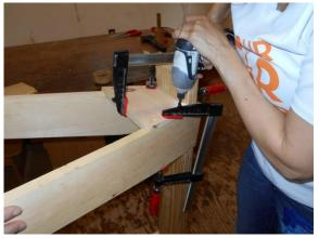
The legs and braces are attached using glue and screws. Shana and Libba then trim the bottoms of the legs to the proper angle and the tops are trimmed flush with the saddle.
